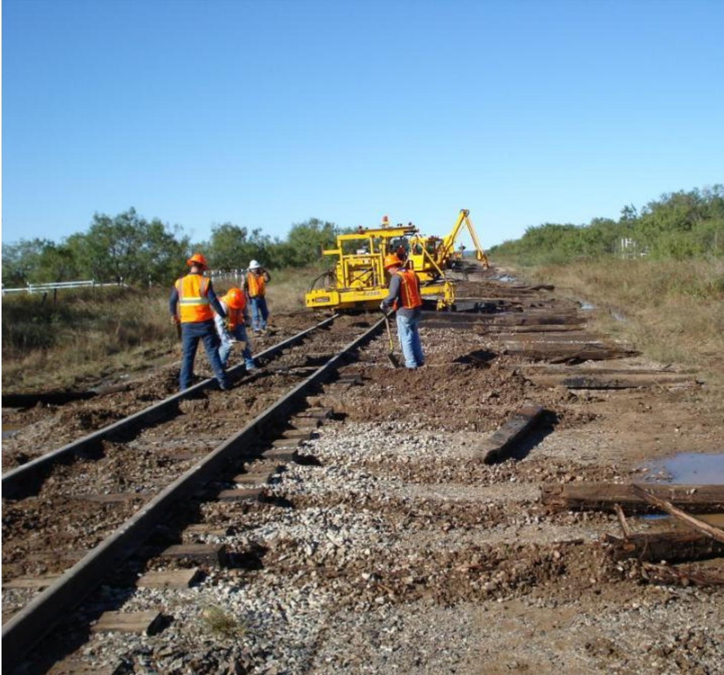
For the rehab work, crews are replacing cross ties, installing ballast, surfacing track and reconstructing grade crossings. All of these tasks are ongoing. The most time-consuming part of the job involves tamping the track to the specified alignment and profile grades.
